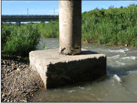
Figure 153. Exposed column footing in stream.
